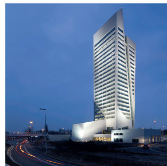
MG Tower Gand, BE
